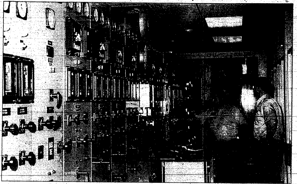
2:30 p.m. - City of Wayne power plant employees Dan Kardell, far left, Keith Doescher, middle, and Gene Hansen work on a wall of dials at the Wayne light plant. Hansen is the power plant supervisor, and Kardell and Doescher are light plant operators. The light plant generators run off diesel, and about 1,300 gallons of fuel is used to run the generators for one hour at full power. (Kim Hansen photo)
